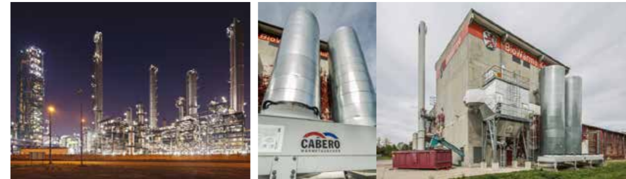
Ecological energy through biomass plants: CABERO systems ensure uninterrupted operation here.
